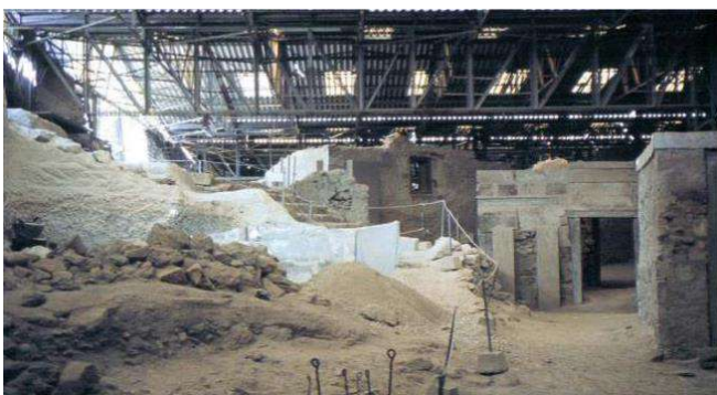
Employing cutting-edge technology of the late 1960s, Marinatos took measures to protect the monuments under a single shelter with a frame of slotted angle steel strips roofed with corrugated asbestos-cement sheeting.
