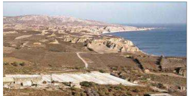
General view of the roof of corrugated asbestos-cement sheeting.
